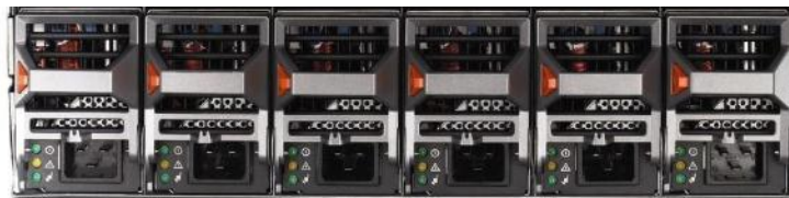
Figure 21. Power Supplies in M1000e
