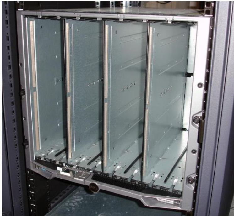
Figure 46. M1000e Mounted in the Rack
